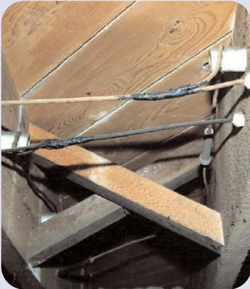
Knob and tube wiring
